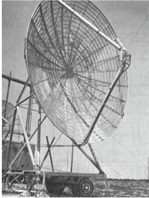
Figure 5-9.—Mobile 30-foot tropospheric-scanner antenna.
